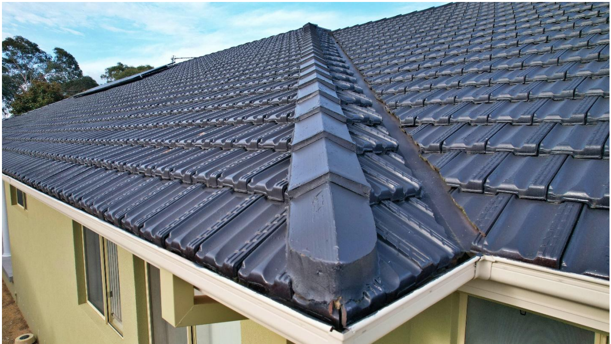
Photo 7 – Whilst less prevalent on this section, there is slight peeling and cracking paint starting to form on the ridge cap and tiles up to the flashing
