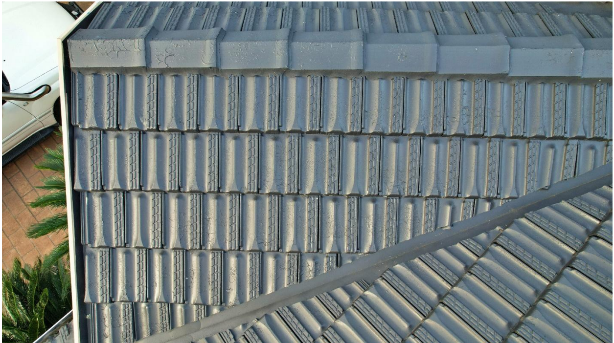
Photo 1 - Peeling, bubbling and cracking paint can be observed along the ridge cap and most tiles
