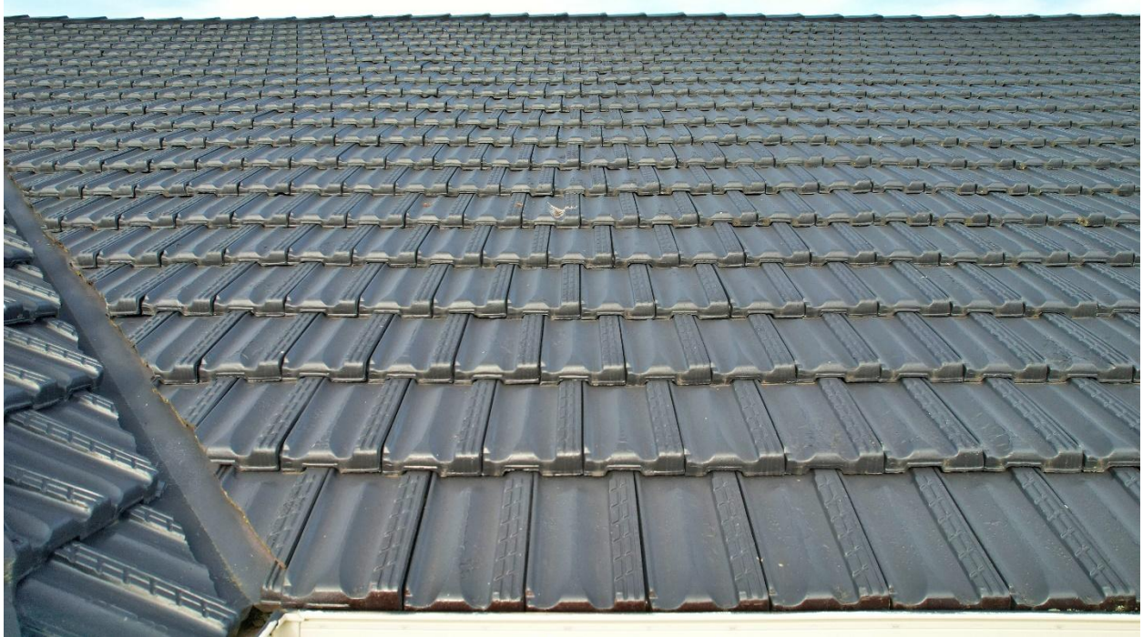
Photo 9 – Whilst less prevalent on this section, there is slight peeling, bubbling and cracking paint starting to form along the ridge cap
