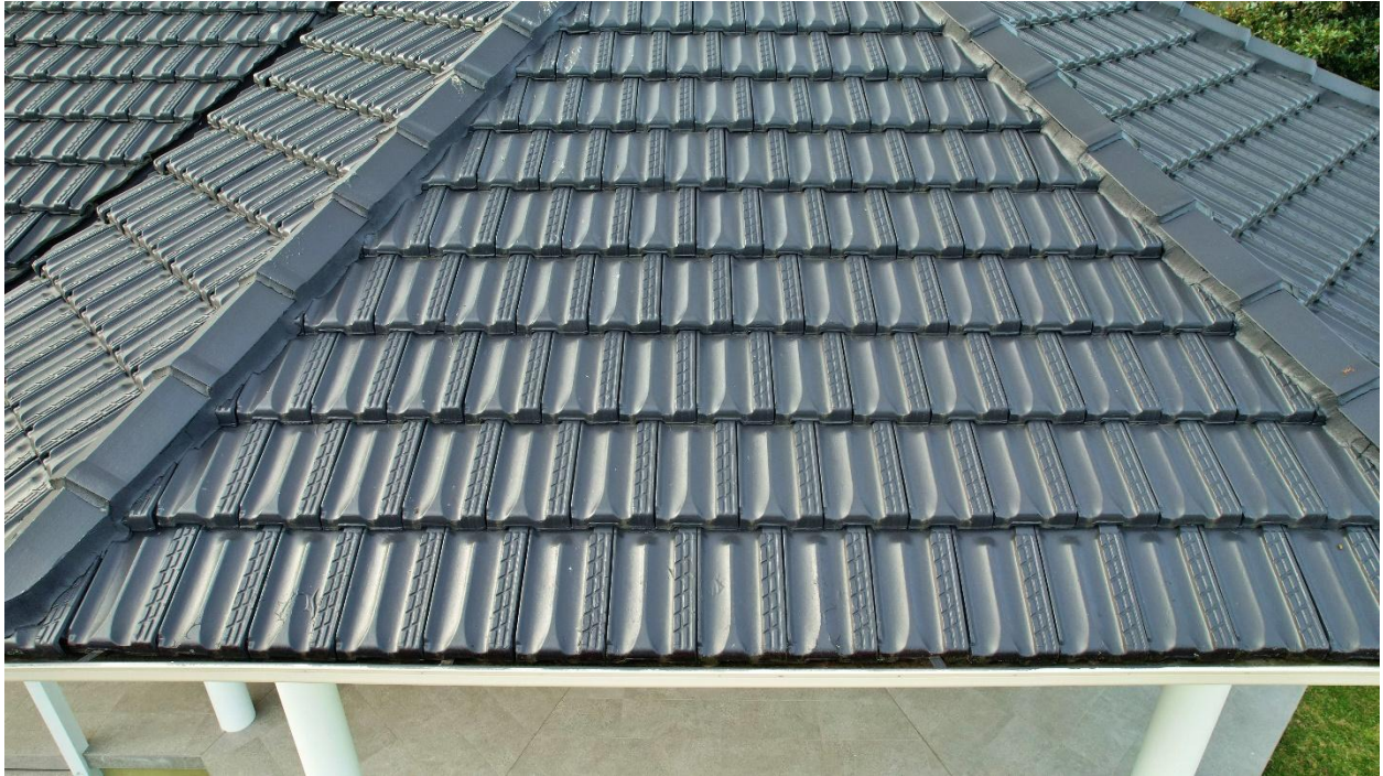
Photo 5 – Whilst less prevalent on this section, there is slight peeling, bubbling and cracking paint starting to form along the ridge cap
