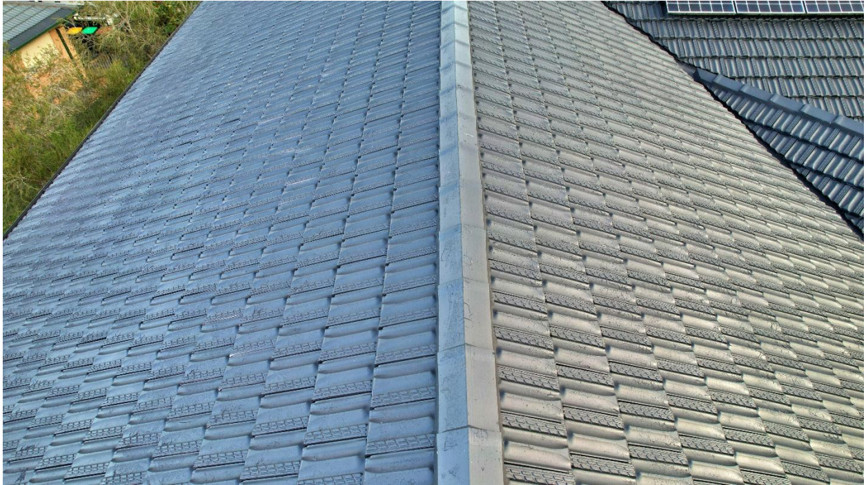
Photo 3 – Paint bubbling and cracking is present along the ridge cap along this section of roof
