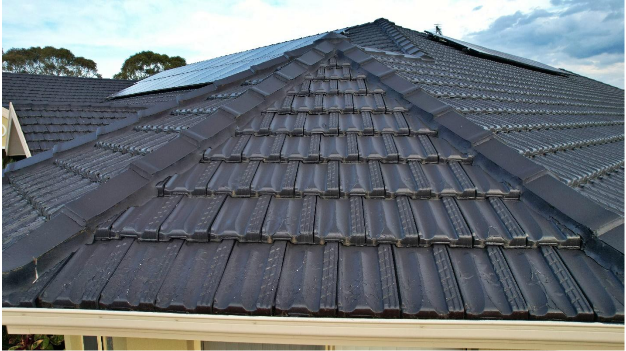
Photo 13 – Top down overview of photos 9-12 showing the extensive paint damage and degradation. This section appears to be the worst on the roof
