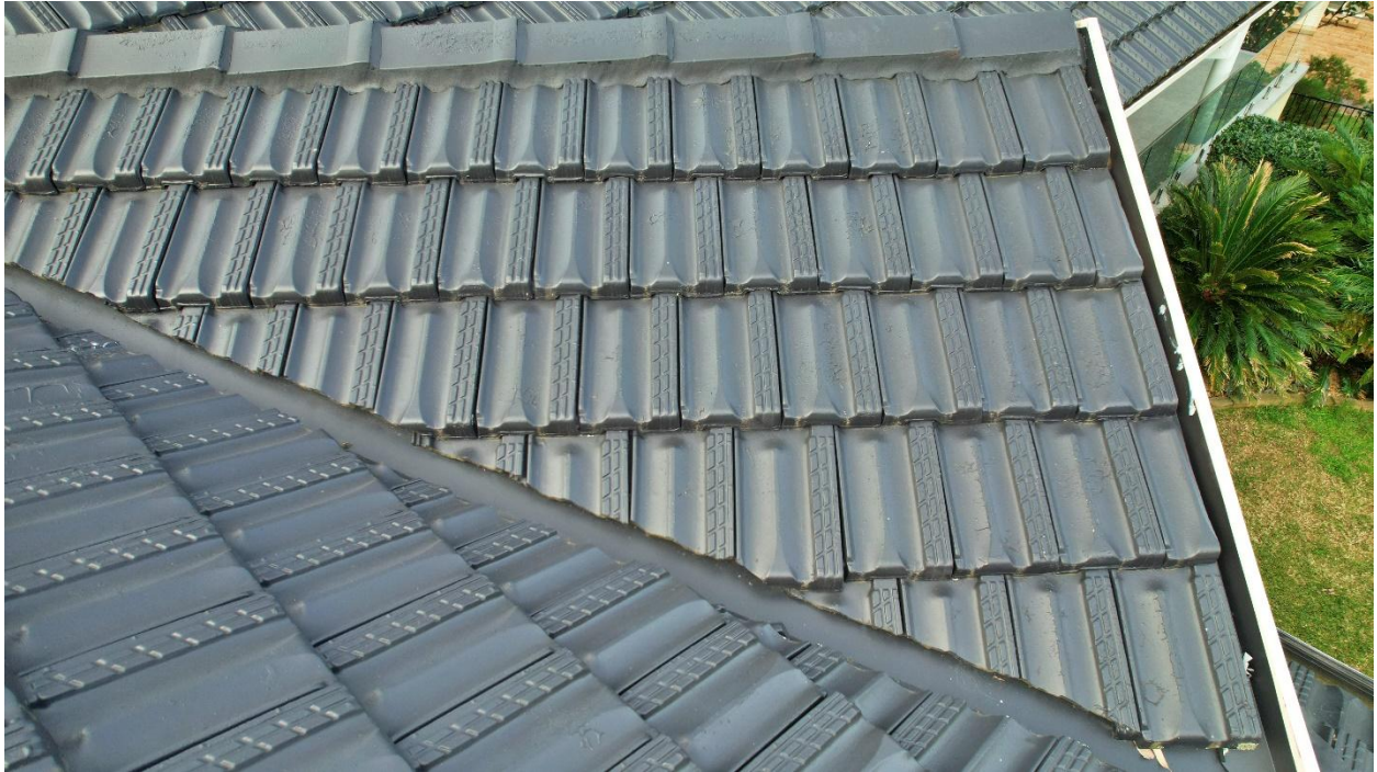
Photo 7 – Close up of roof section along the flashing, showing peeling, bubbling and cracking paint on tiles and the ridge capping
