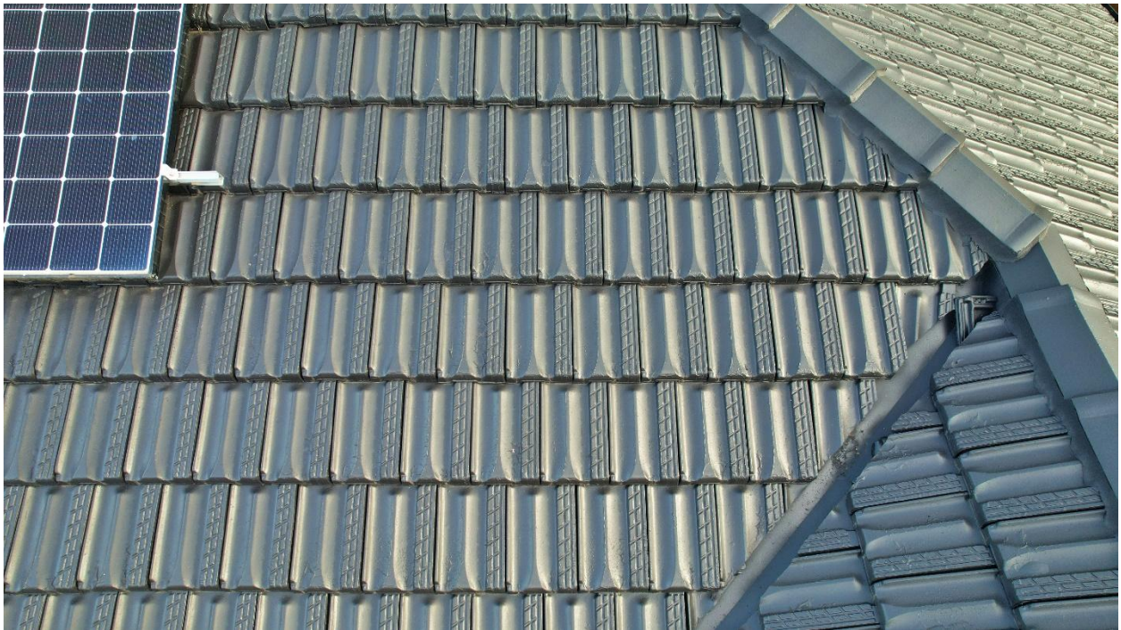
Photo 15 – Close up of roof section, showing peeling, bubbling and cracking. Extensive damage and degradations are observed around the solar .
