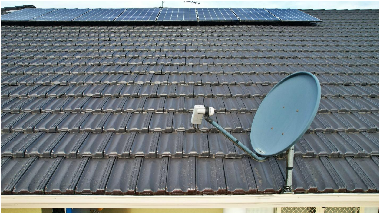
Photo 5 - Close up of roof section along the gutter line, showing peeling, bubbling and cracking paint which extends from the gutter to solar panels
