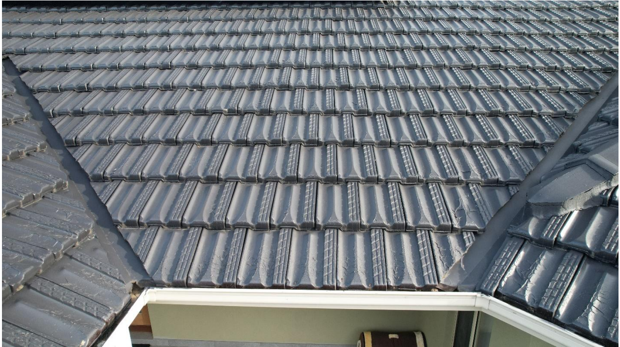
Photo 9 - Close up of roof section along the gutter line, showing peeling, bubbling and cracking paint
