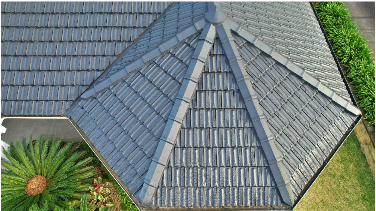
Photo 13 – Top down overview of photos 9-12 showing the extensive paint damage and degradation. This section appears to be the worst on the roof
