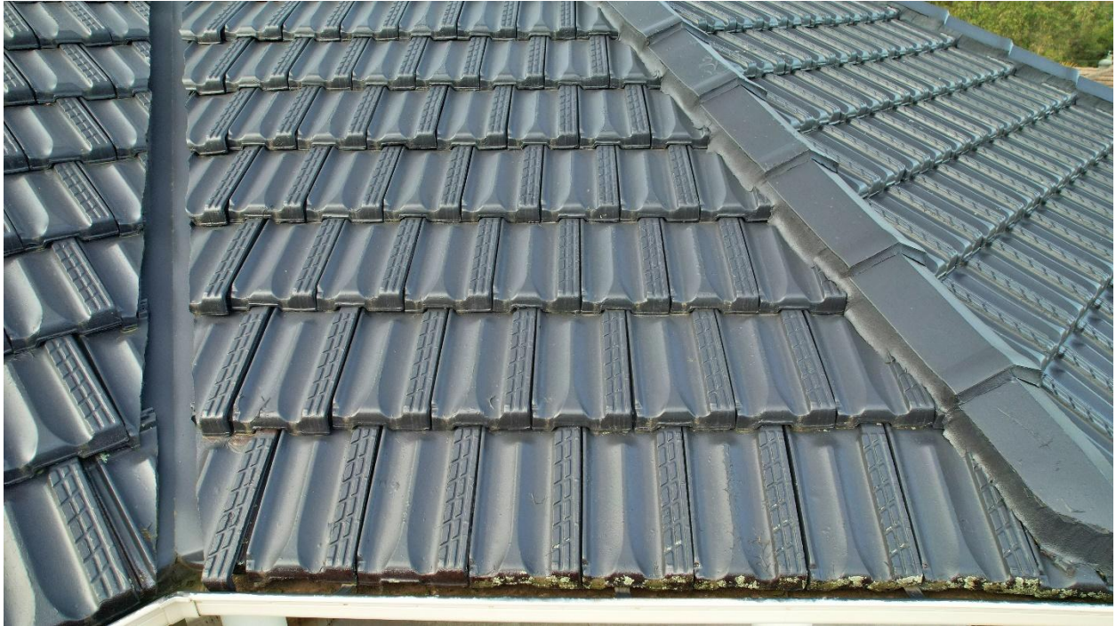
Photo 3 – Whilst less prevalent on this section, there is slight peeling, bubbling and cracking paint starting to form along the ridge cap
