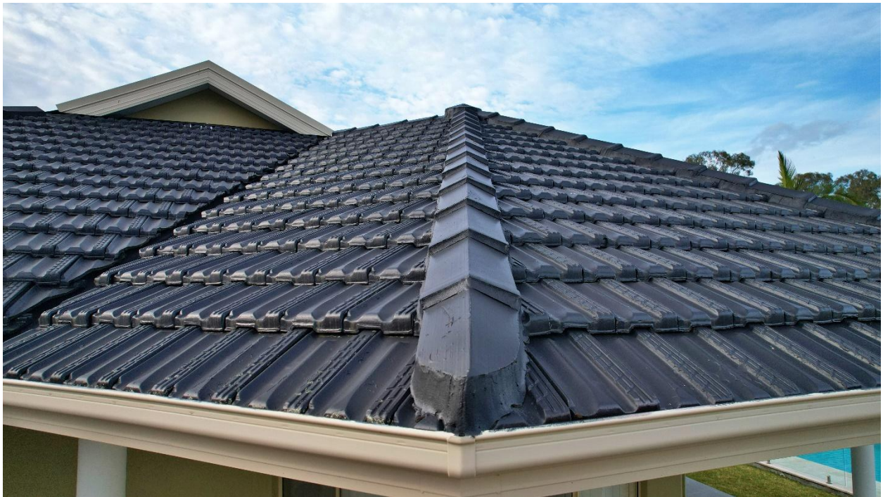
Photo 3 – Whilst less prevalent on this section, there is slight peeling, bubbling and cracking paint starting to form along the ridge cap
