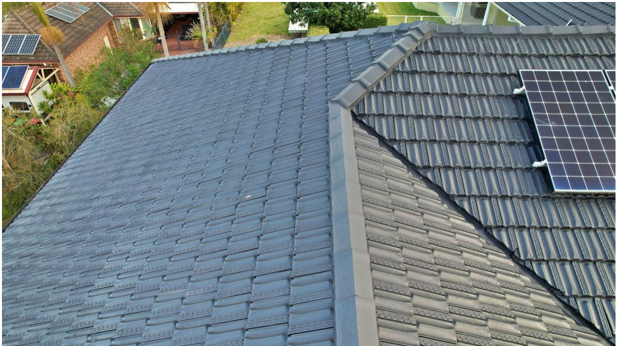
Photo 3 – Paint bubbling and cracking is present along the ridge cap along this section of roof
