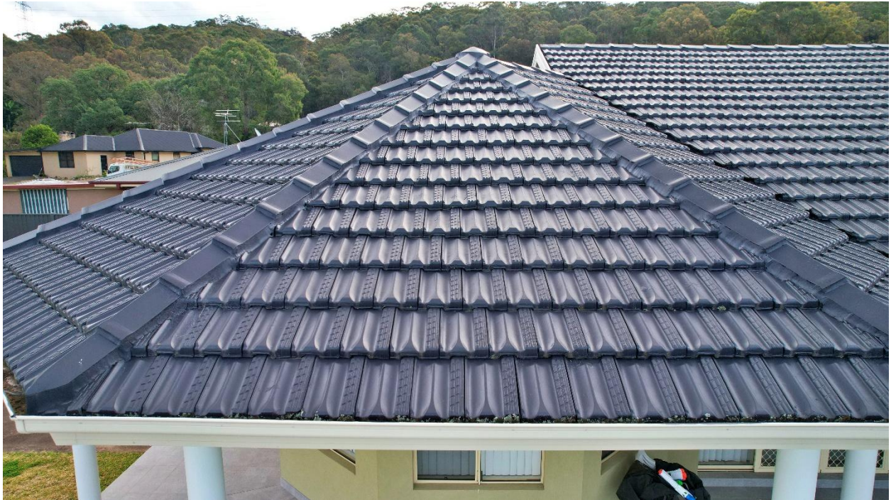
Photo 5 – Whilst less prevalent on this section, there is slight peeling, bubbling and cracking paint starting to form along the ridge cap
