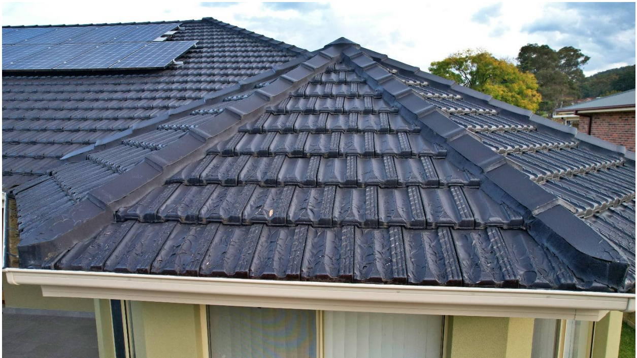
Photo 11 - Close up of the gutterline and ridge cap. Peeling, bubbling and cracking is very bad in the section of the roof
