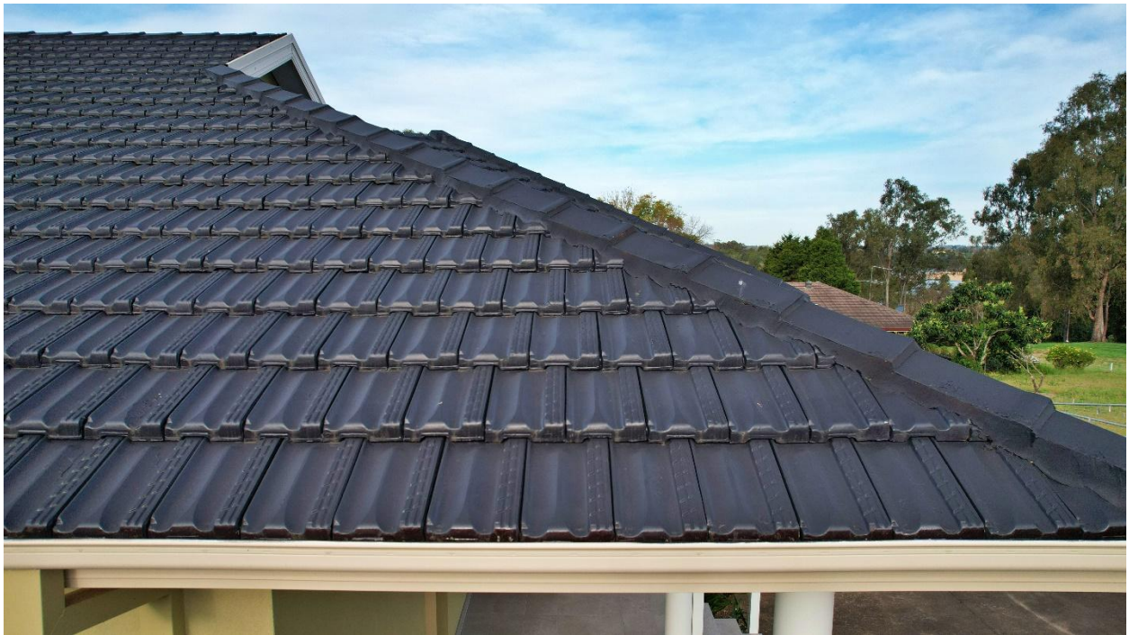
Photo 9 – Whilst less prevalent on this section, there is slight peeling, bubbling and cracking paint starting to form along the ridge cap
