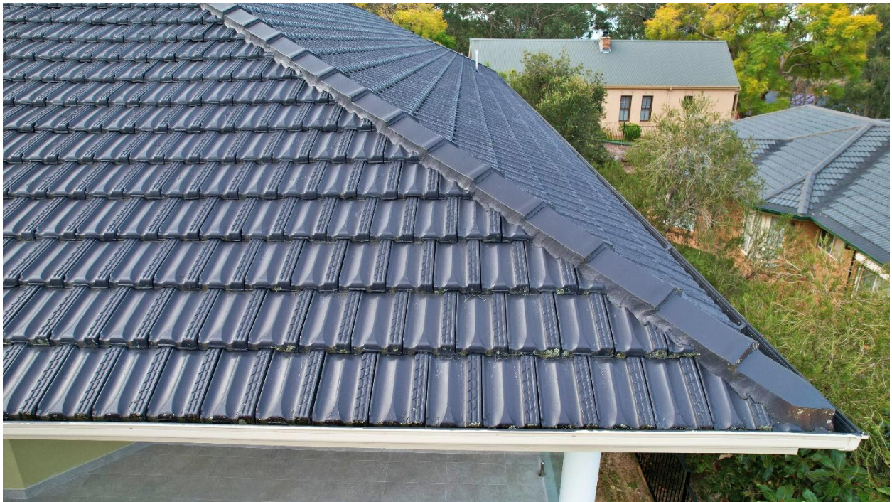
Photo 3 – Whilst less prevalent on this section, there is slight peeling, bubbling and cracking paint starting to form along the gutter line
