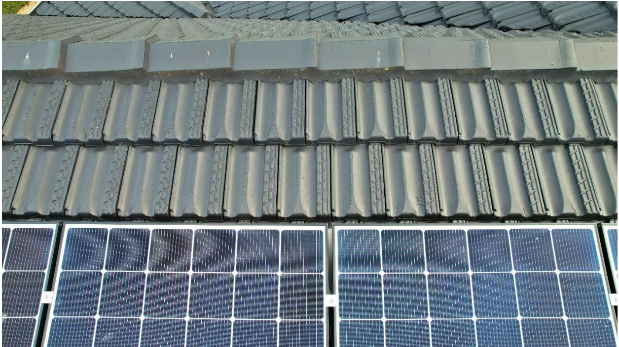
Photo 3 - Close up of roof section along the solar panel and ridge capping, showing peeling, bubbling and cracking paint on tiles is extensive
