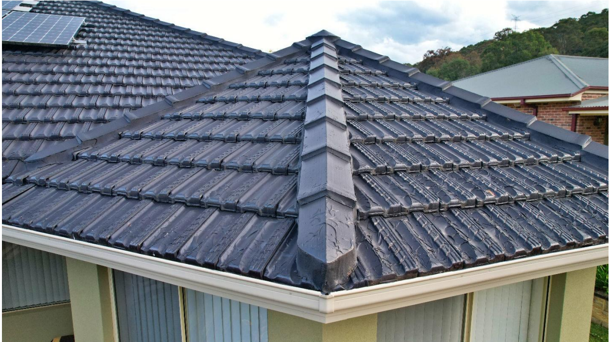
Photo 11 - Close up of the gutterline and ridge cap. Peeling, bubbling and cracking is very bad in the section of the roof
