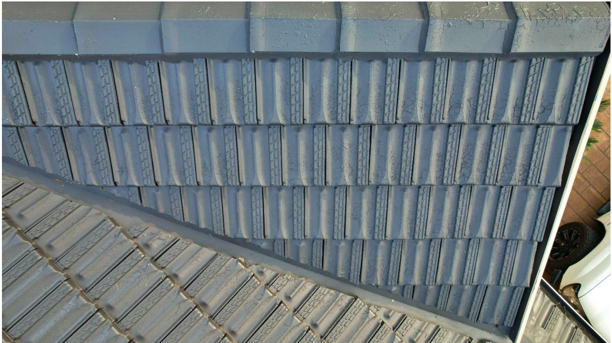
Photo 3 – Peeling and cracking paint can be observed along the ridge cap and most tiles
