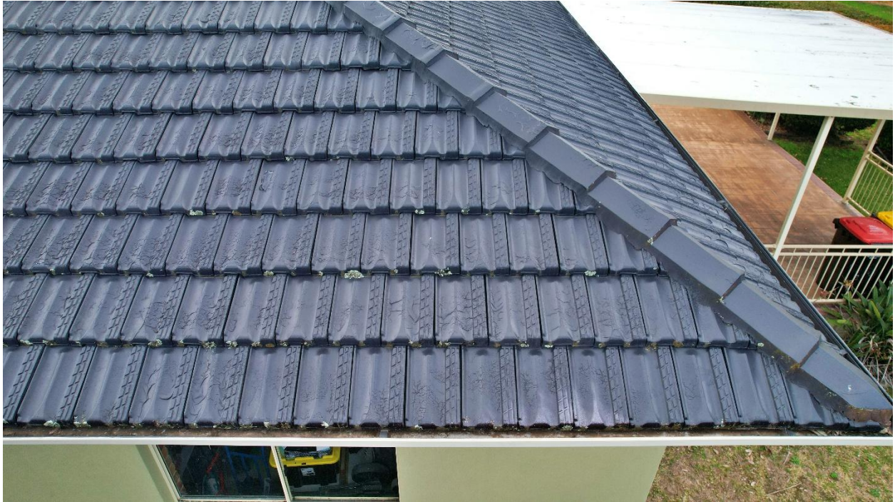
Photo 9 - Top down overview of photos 4-6 showing the extensive paint damage and degradation. This section appears to be quite damaged
