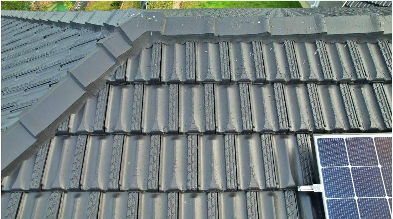
Photo 1 - Close up of roof section along the solar panel and ridge capping, showing peeling, bubbling and cracking paint on tiles is extensive
