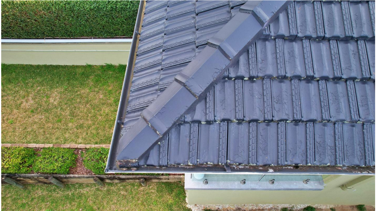
Photo 3 - Close up of roof section along the gutter line, showing peeling, bubbling and cracking paint
