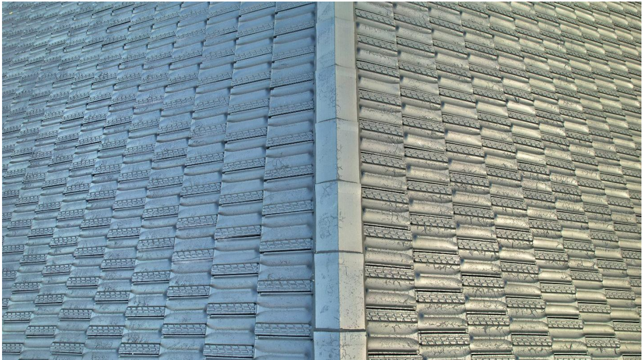
Photo 1 – Paint peeling and cracking is present along the ridge cap along this section of roof
