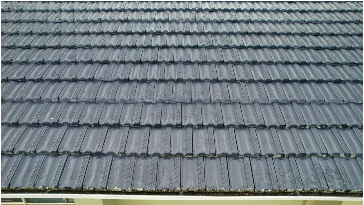
Photo 3 - Close up of roof section along the gutter line, showing peeling, bubbling and cracking paint
