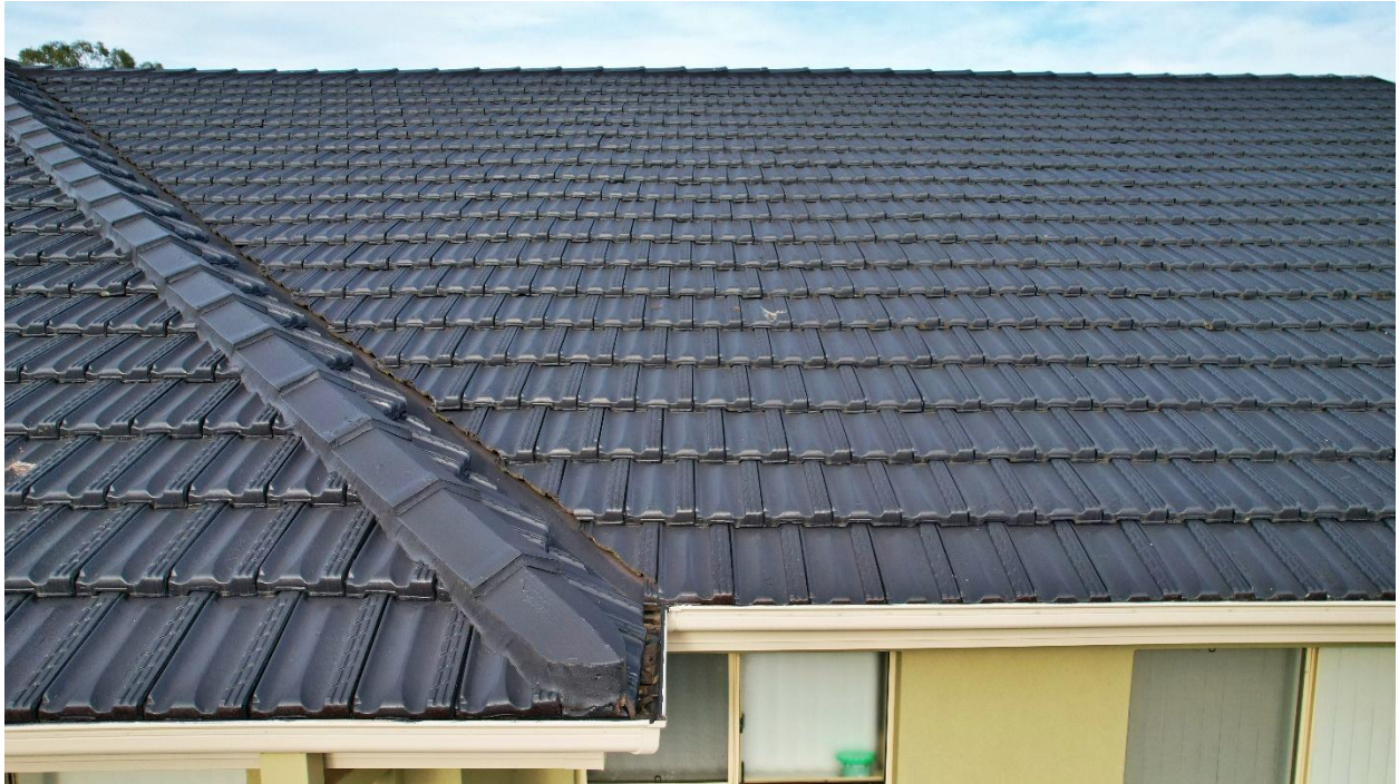
Photo 7 – Whilst less prevalent on this section, there is slight peeling and cracking paint starting to form on the ridge cap and tiles up to the flashing
