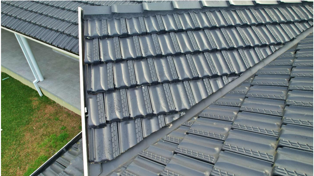
Photo 7 – Close up of roof section along the flashing, showing peeling, bubbling and cracking paint on tiles and the ridge capping
