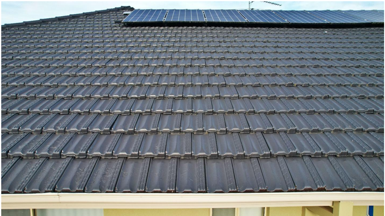
Photo 3 - Close up of roof section along the gutter line, showing bubbling and cracking paint which extends from the gutter to solar panels
