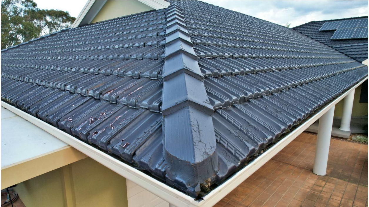
Photo 7 – Gable close up showing the paint peeling, bubbling and cracking is constant up to the gable and flashing
