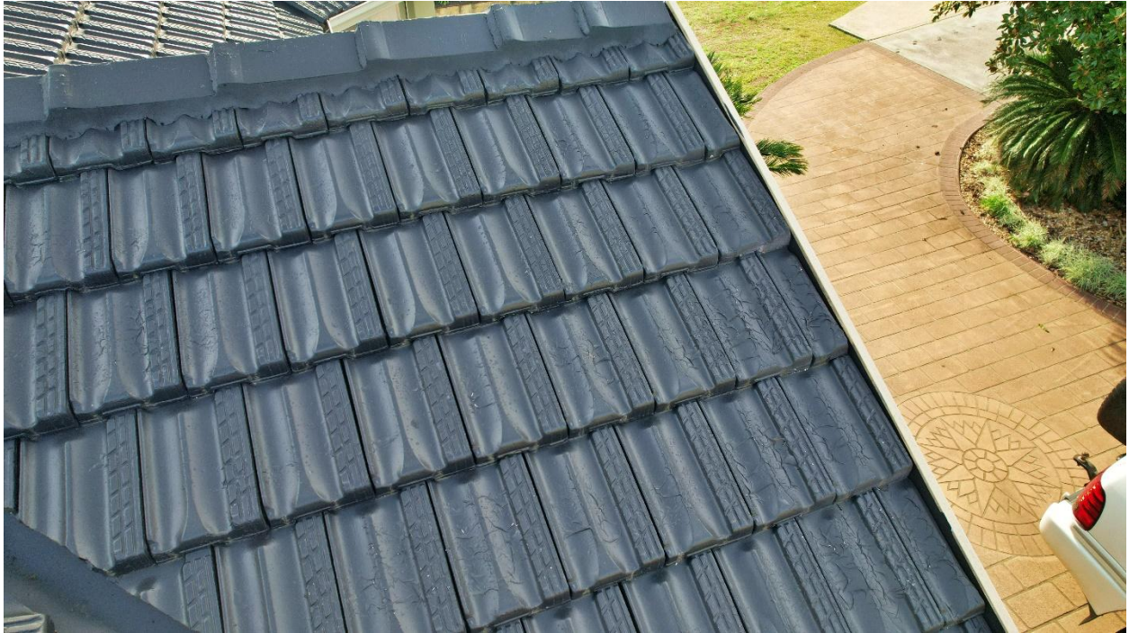
Photo 7 - Close up of roof section, showing, peeling, bubbling and cracking paint
