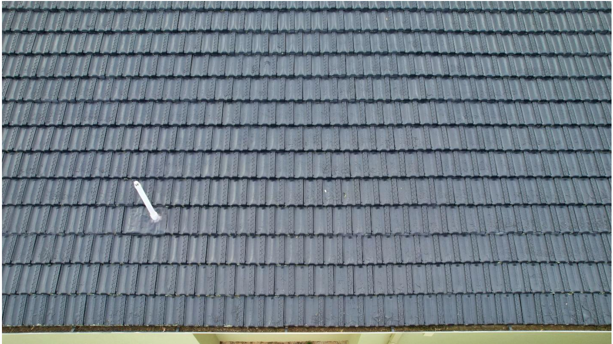
Photo 9 - Top down overview of photos 4-6 showing the extensive paint damage and degradation. This section appears to be quite damaged
