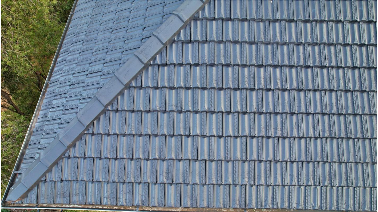
Photo 5 – Right hand side of the roof section. In the photo, the peeling and bubbling is heavily present along the gutterline to ridge cap
