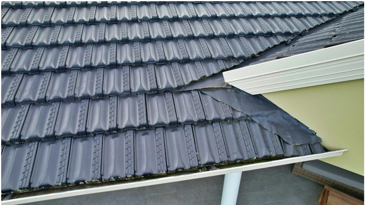
Photo 5 – Whilst less prevalent on this section, there is slight peeling, bubbling and cracking paint starting to form along the gutter line
