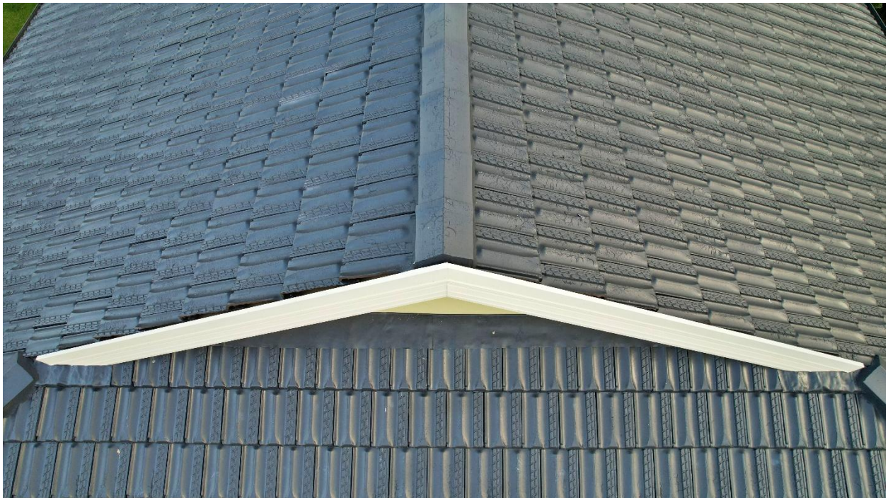
Photo 7 – Gable close up showing the paint peeling, bubbling and cracking is constant up to the gable and flashing
