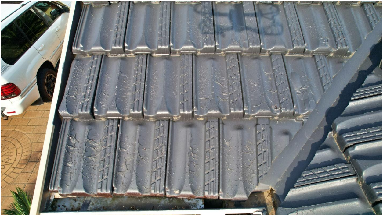
Photo 7 - Close up of roof section, showing, peeling, bubbling and cracking paint
