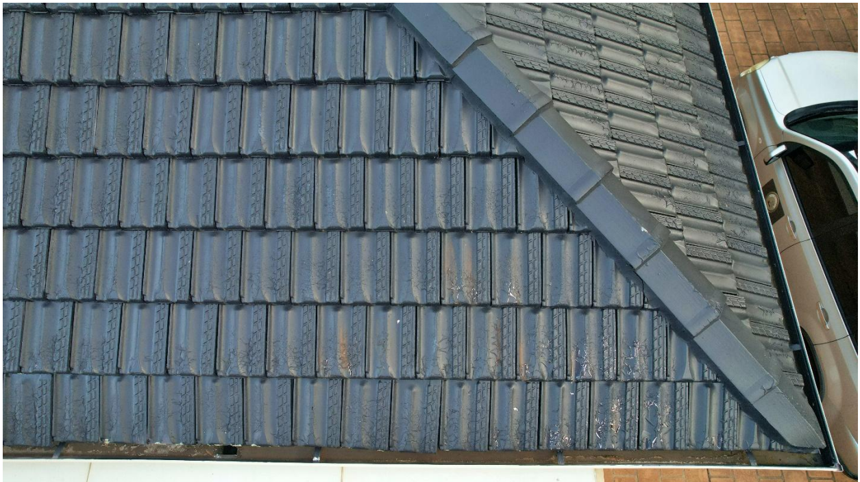
Photo 5 – Right hand side of the roof section. In the photo, the peeling and bubbling is heavily present along the gutterline to ridge cap
