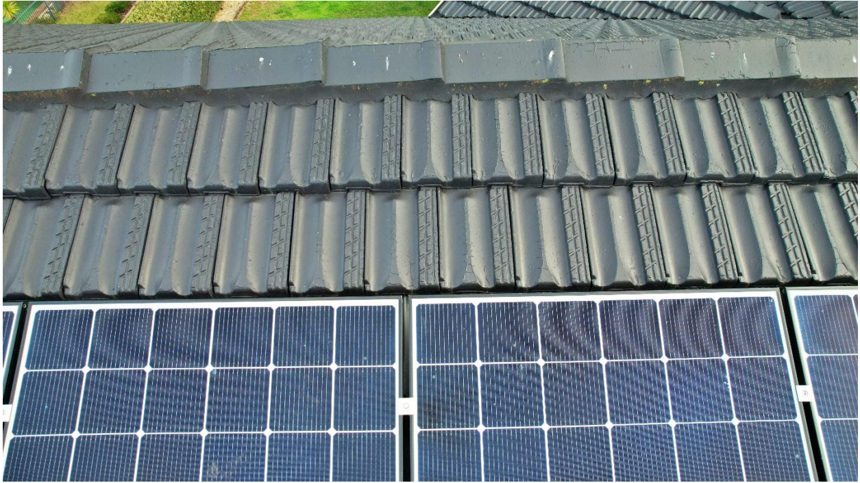
Photo 3 - Close up of roof section along the solar panel and ridge capping, showing peeling, bubbling and cracking paint on tiles is extensive
